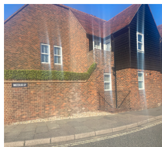
Waterloo Road Depaving
