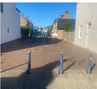
Warwick Road/Regent Street Depaving
