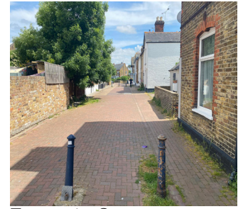
Fountain Street DePaving
