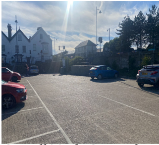
Gorrell Tank Car Park Addition of rain gardens, changed mowing, green roofs
